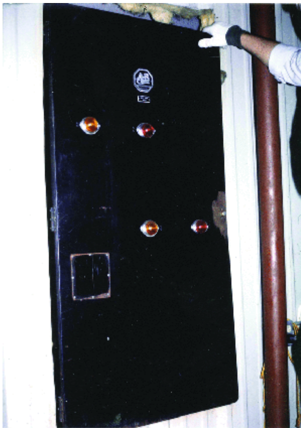
Figure 2. Electrical control panel used as a secret access door to the hidden storage rooms with tanks for liquid beet sugar.
